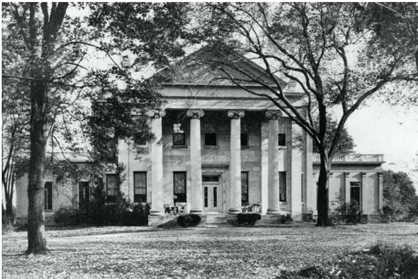
Fig. 9 Mercer Manor 410 Mercer Road
