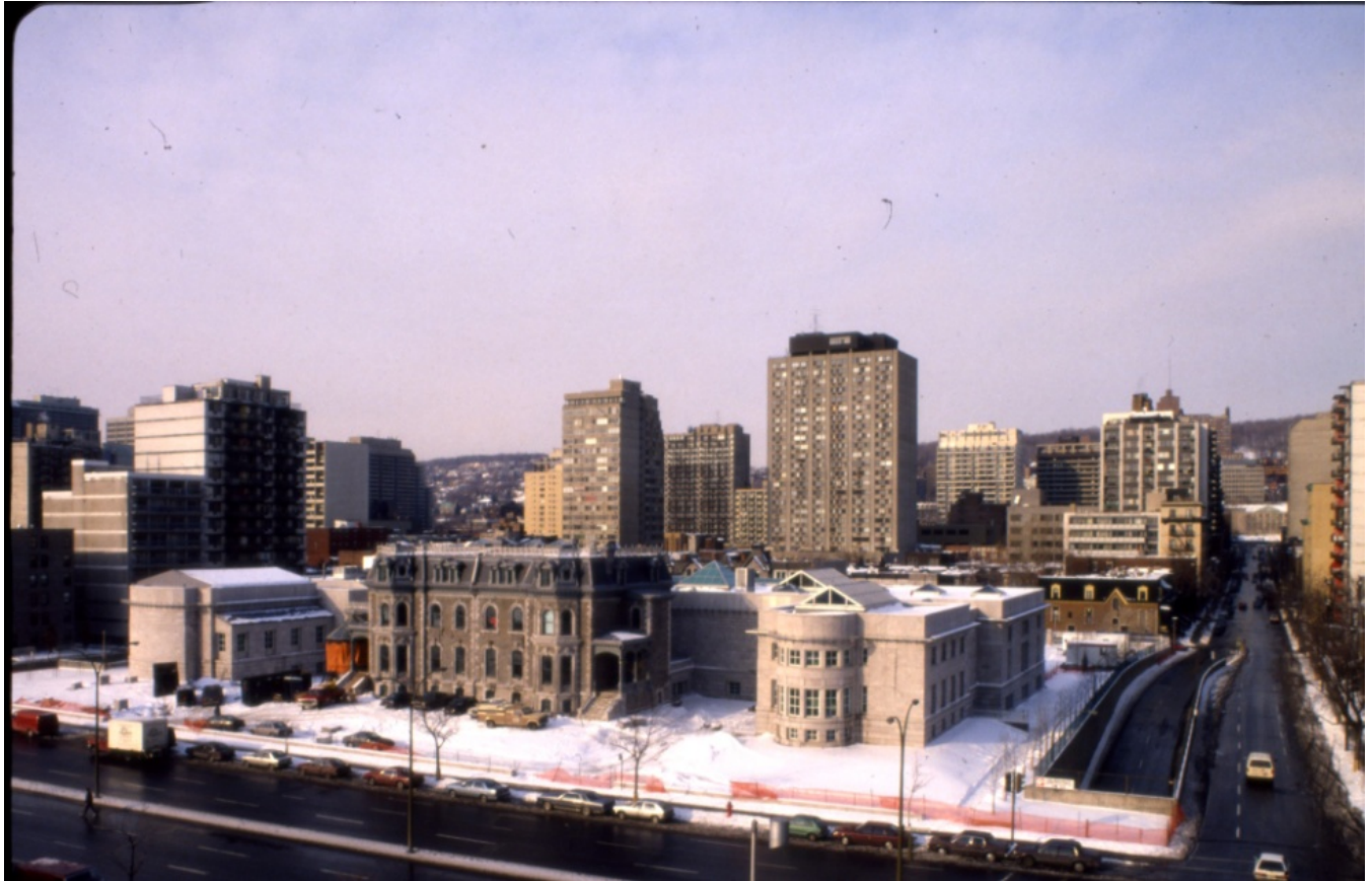
Fig. 24 Canadian Centre for Architecture, south façade. Montreal
