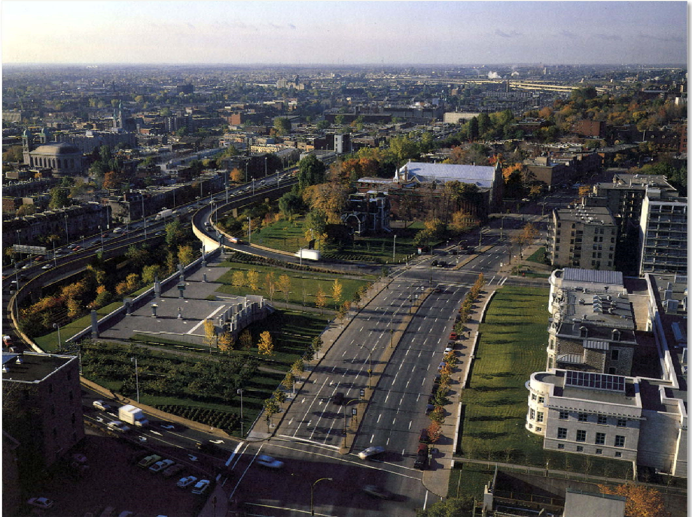
Fig. 27 Air view toward southwest of Canadian Centre for Architecture and garden
