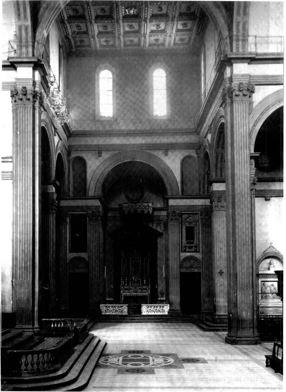
Fig. 21. View of north transept. San Lorenzo, Florence (photo: Brogi 26240).
