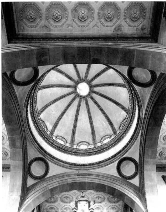
Fig. 30. View of the dome. Santo Spirito, Florence (photo: Alinari 62653).
